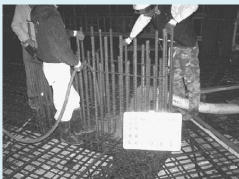
(a) Compacting concrete
