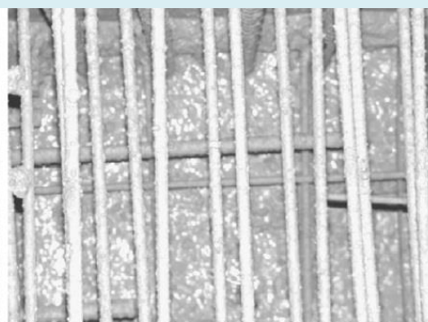
(b) Concrete inside a column
